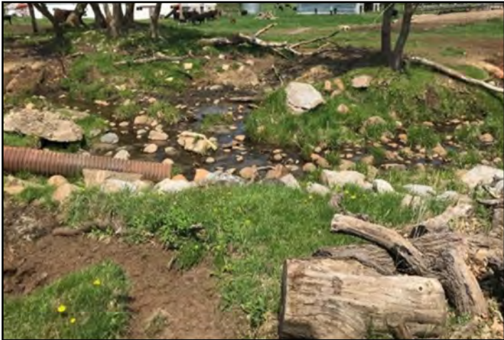
Photo A above shows the erosion and much disturbance where the cattle crossed the stream from one pasture to the next. Photo B is taken from the same vantage point, after construction, showing the restricted cattle—cross area with an appropriately sized culvert below the gravel pad. Photo C , below left, shows other areas of the stream void of vegetation, prior to the project, where cattle congregated for shade and water. Photo D , bottom right, shows the healing process of revegetation now that the cattle are fenced off from this area. Public Works should see benefits to the culvert under the county road in the years to come.
