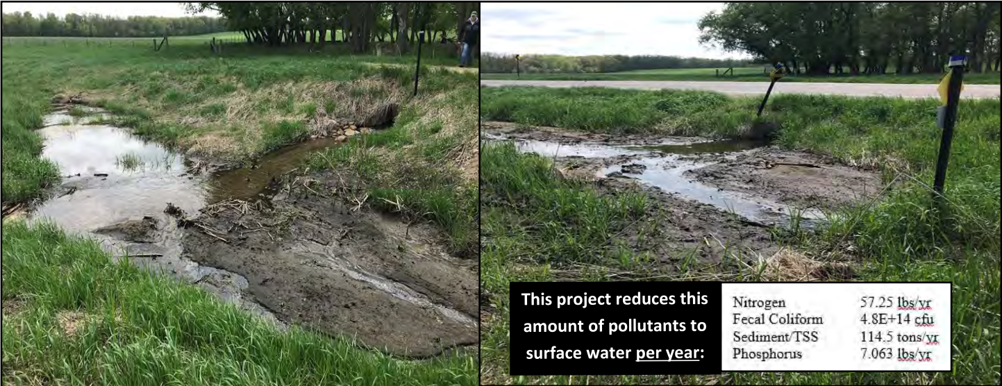
Photos above indicate the volume of sediment building up in the county road ditch on both the east and west sides of the road every year. The problem was caused by erosion due to lack of vegetation along the streambank and cattle disturbance upstream.
