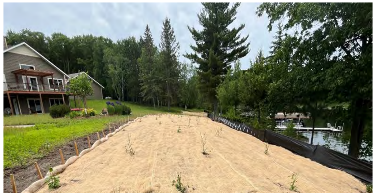
Native Shoreland buffer project being installed to replace turf grass lawn on Pine Island Lake, Todd County
