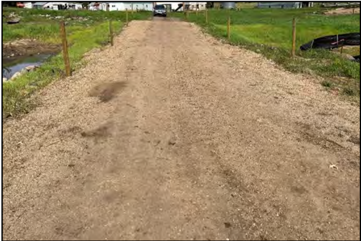
Photo A above shows the erosion and much disturbance where the cattle crossed the stream from one pasture to the next. Photo B is taken from the same vantage point, after construction, showing the restricted cattle—cross area with an appropriately sized culvert below the gravel pad. Photo C , below left, shows other areas of the stream void of vegetation, prior to the project, where cattle congregated for shade and water. Photo D , bottom right, shows the healing process of revegetation now that the cattle are fenced off from this area. Public Works should see benefits to the culvert under the county road in the years to come.
