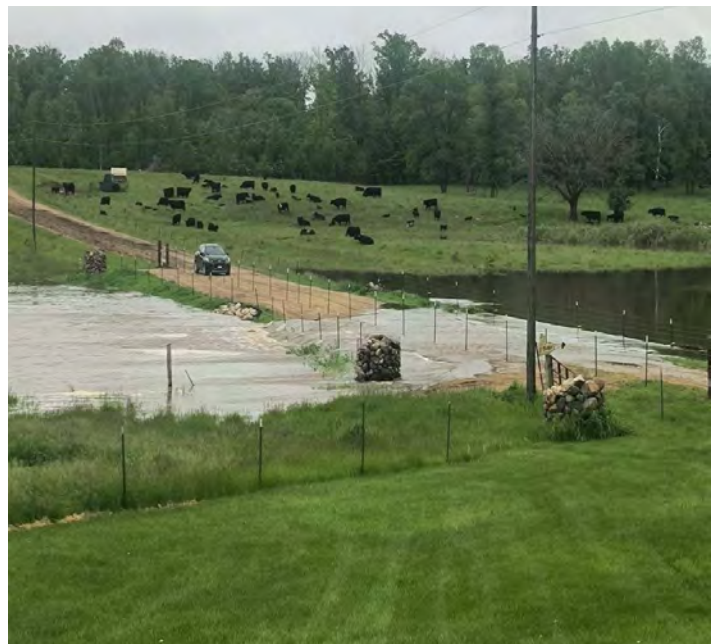
Above, last erosion blanket laid and stormwater controls in place just before the flooding event. Below, both pictures show the receding flood waters of the Partridge River remaining overtop the newly installed cattle crossing.
