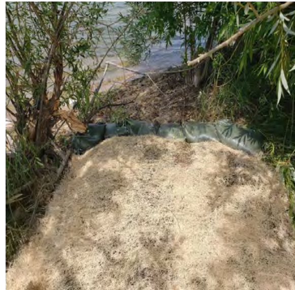
Photo: The inlet to Fairy Lake was stabilized at the culvert under County 11 using tuff reinforcement mat and an erosion control blanket.
